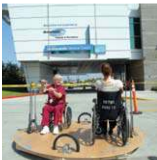
From top to bottom: 1) Two future playground users visit the construction site; 2) OHMMHS students exhibit a popsicle-stick model of a universally accessible merry-go-round they designed; 3) Cal State mechanical engineering students test some of the mechanisms to be used in the prototype design; 4) wood-frame mockup of the base; 5) prototype merry-go-round gets taken for a "test spin" by LAOH staff members.
