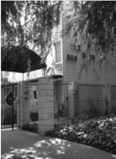
The Everychild grant is being used to purchase this Pasadena apartment building, eventual home to 28 emancipated foster youth.
